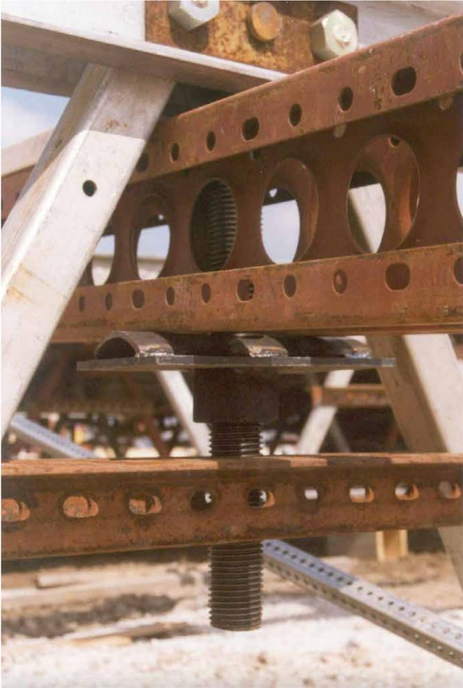
*Symons Soldier Beams and a custom washer with a curved surface were part of the support assembly that allowed the tables to achieve a slope.*
