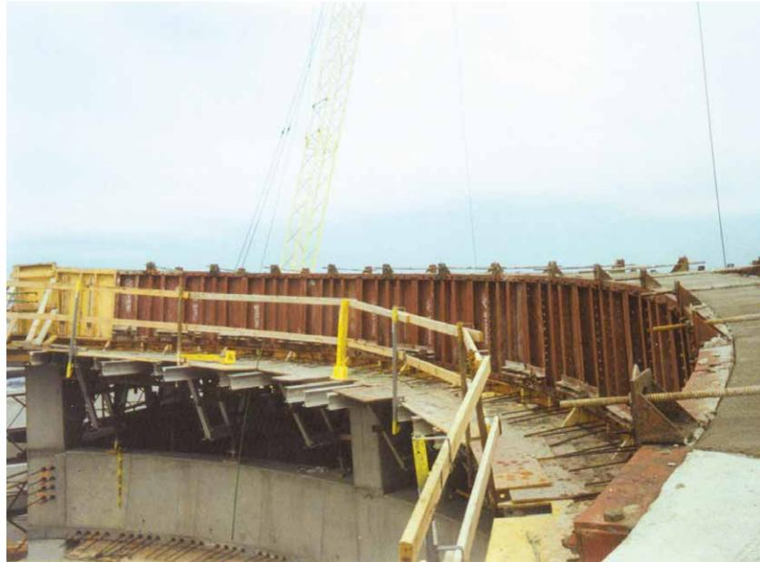
*Flex-Form panels were used to form the curved 4' high barrier wall.*
